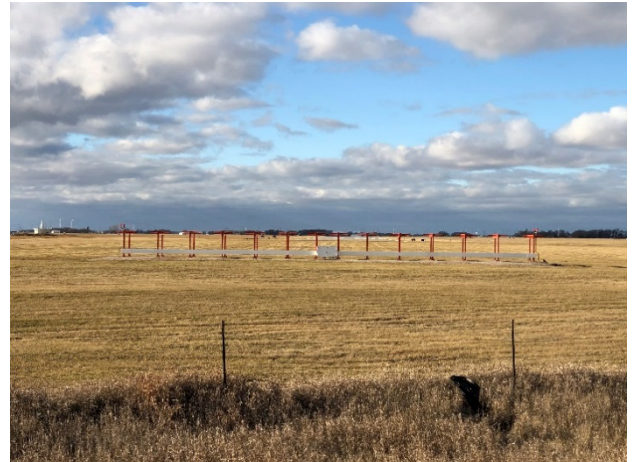
Localizer Antenna Array
