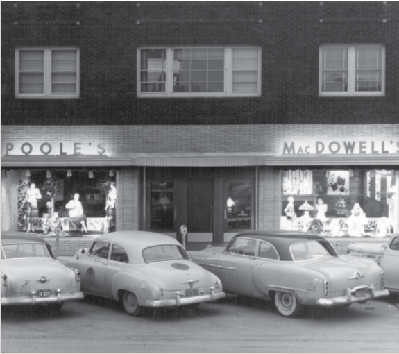
Historic signage on the Poole Building (528 Grand) utilized illuminated, individual letters. Notice the light is concentrated on the letters only, and the letters project up from a simple base. They do not alter the facade because they are not attached to a board which is then attached to the building.
